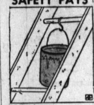
A POT HOOK should be used when working from a ladder. The Institute for Safer Living attributes many painful acci-dents to falling paint buckets.
