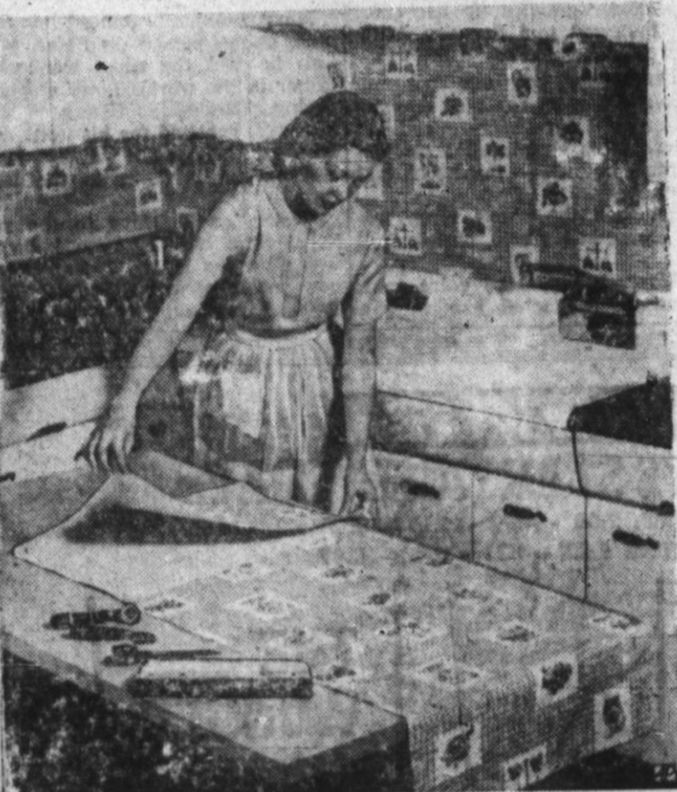
PREPARE several strips ahead of time as professionals do. Brush paste evenly and fold two-thirds, then one-third.
