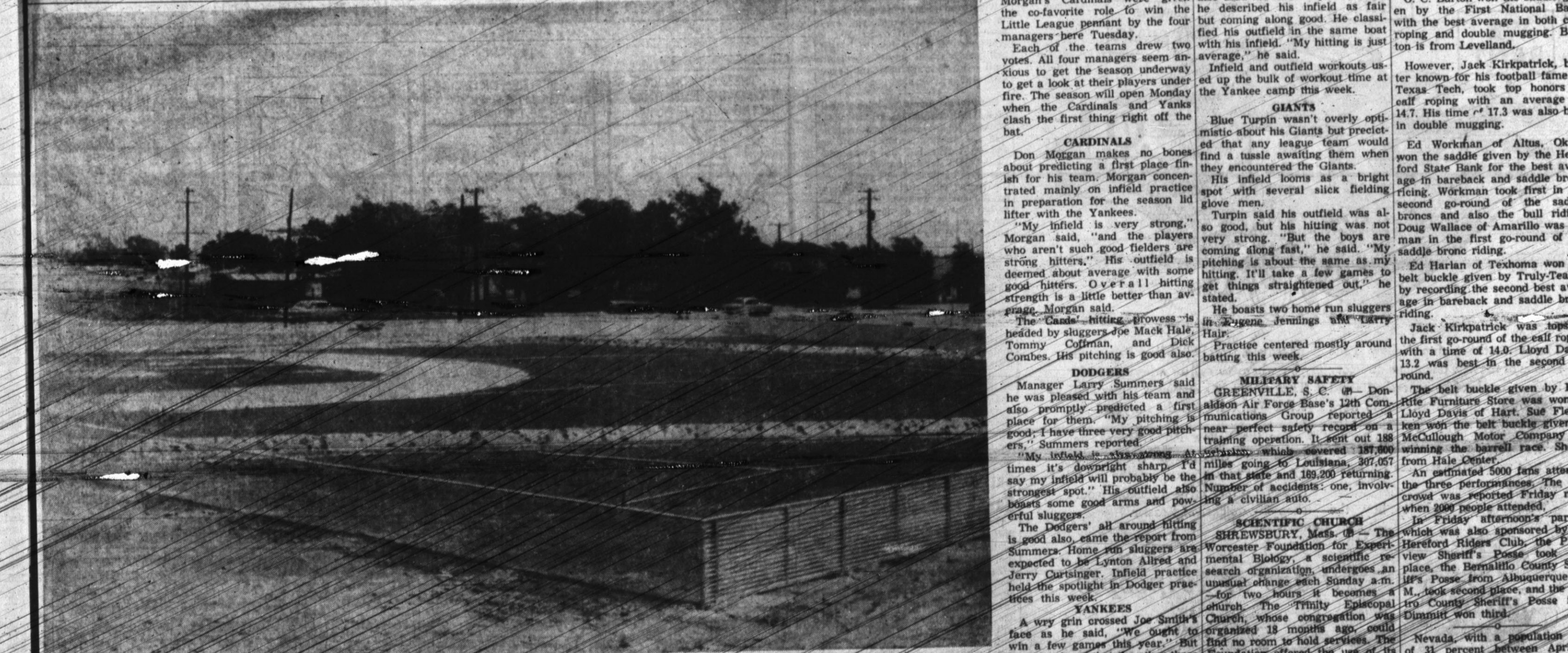
NEARS COMPLETION—Nearing completion is Hereford's new Little League Baseball Park. The Jaycoes, who are doing the work on the park, reported this week that it should be completed by the time the season starts Monday, June 11. The metal outfield fence will be painted green, construction workers said, to kill the glare of the sun.
