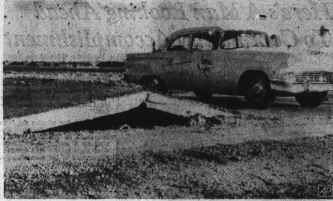
HEAT BUCKLES HIGHWAY—This section of little or no relief in sight to dent the Texas US Highway 67 was buckled by intense heat heat wave. (AP Photo) as temperature soared to 107 degrees with
