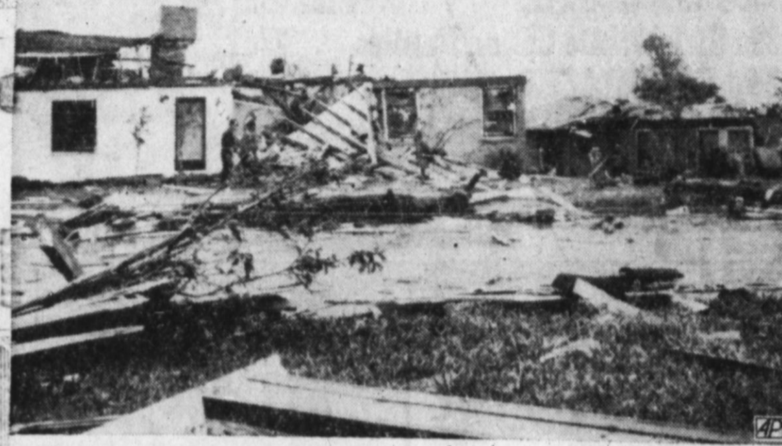
HOMES DESTROYED BY TORNADO—A part of the 25 homes destroyed when a tornado tore through Tyler are shown here. The twister also damaged two schools and some other buildings. (AP Photo)
