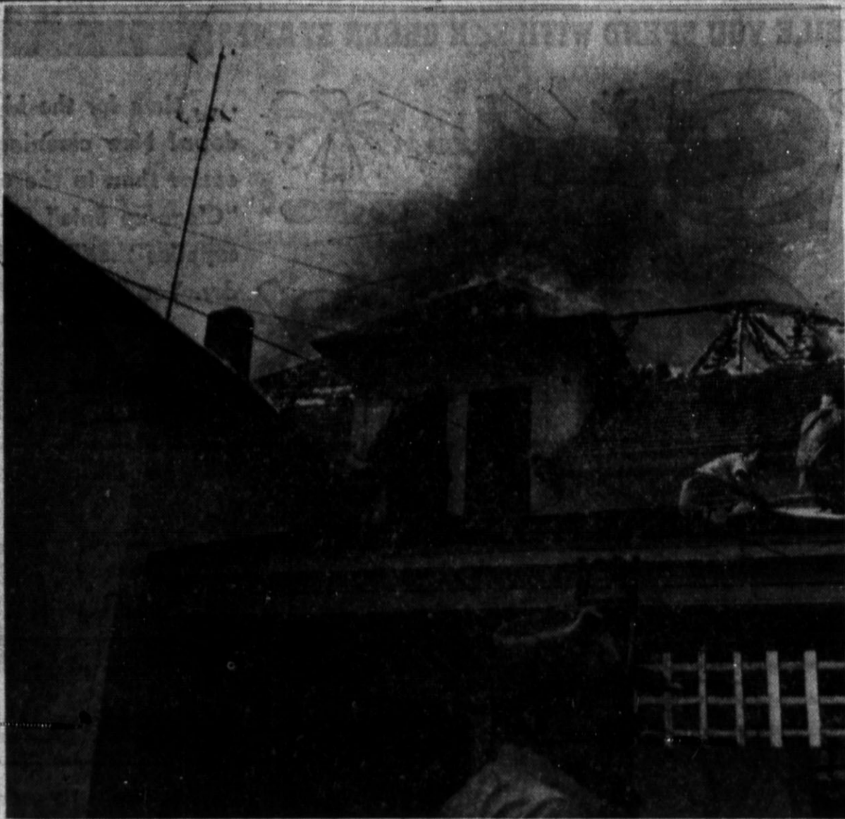
HEREFORD VOLUNTEER FIRE DEPARTMENT Extensive damage resulted from the fire extinguished a fire which gutted the upper section of the home of Mr. and Mrs. Harley Davis, 709 Grand, Thursday afternoon, on the roof, in the attic and on the second floor. Water damaged much of the ground floor portion. (Staff Photo)
