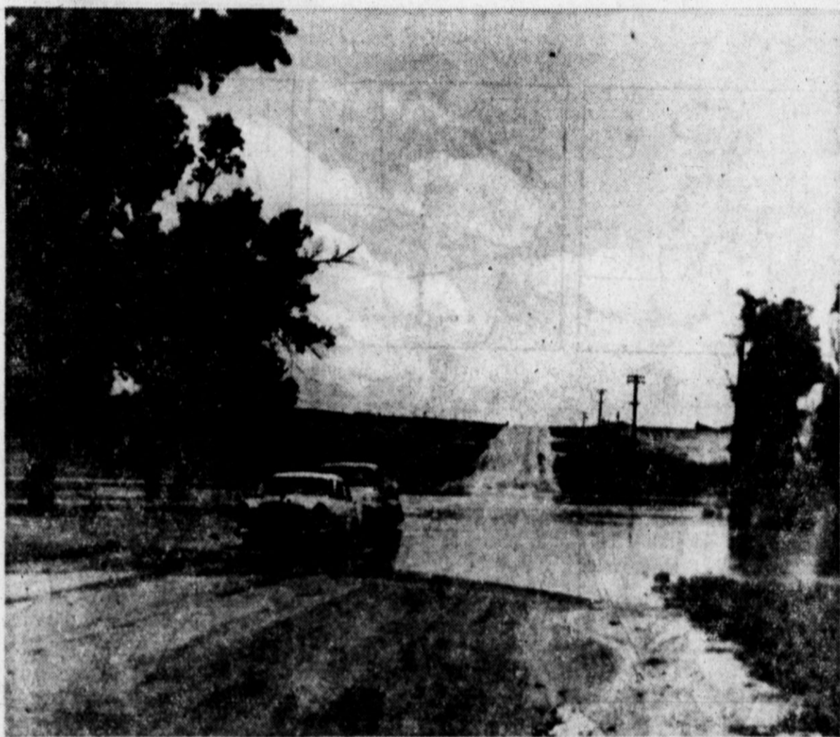
TIERRA BLANCA CREEK became a small river its bank and covered the paved road, stalled Tuesday and Wednesday after heavy rains. ing some vehicles and causing drivers to Southwest of Hereford, the creek jumped detour. (Staff Photo)
