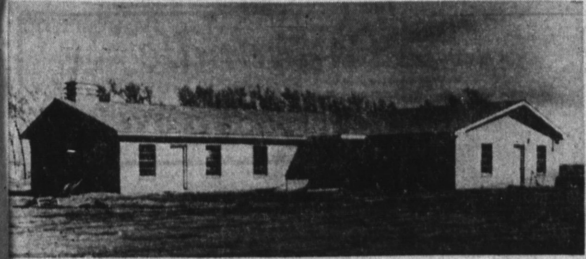
FIRST SERVICES were held Sunday in the new building of the Westway Baptist Church. Regular services are held at 10 a. m. and 6:30 p. m. The brick structure is located on the south side of Harrison Highway about five miles west of Hereford. (Staff Photo)
