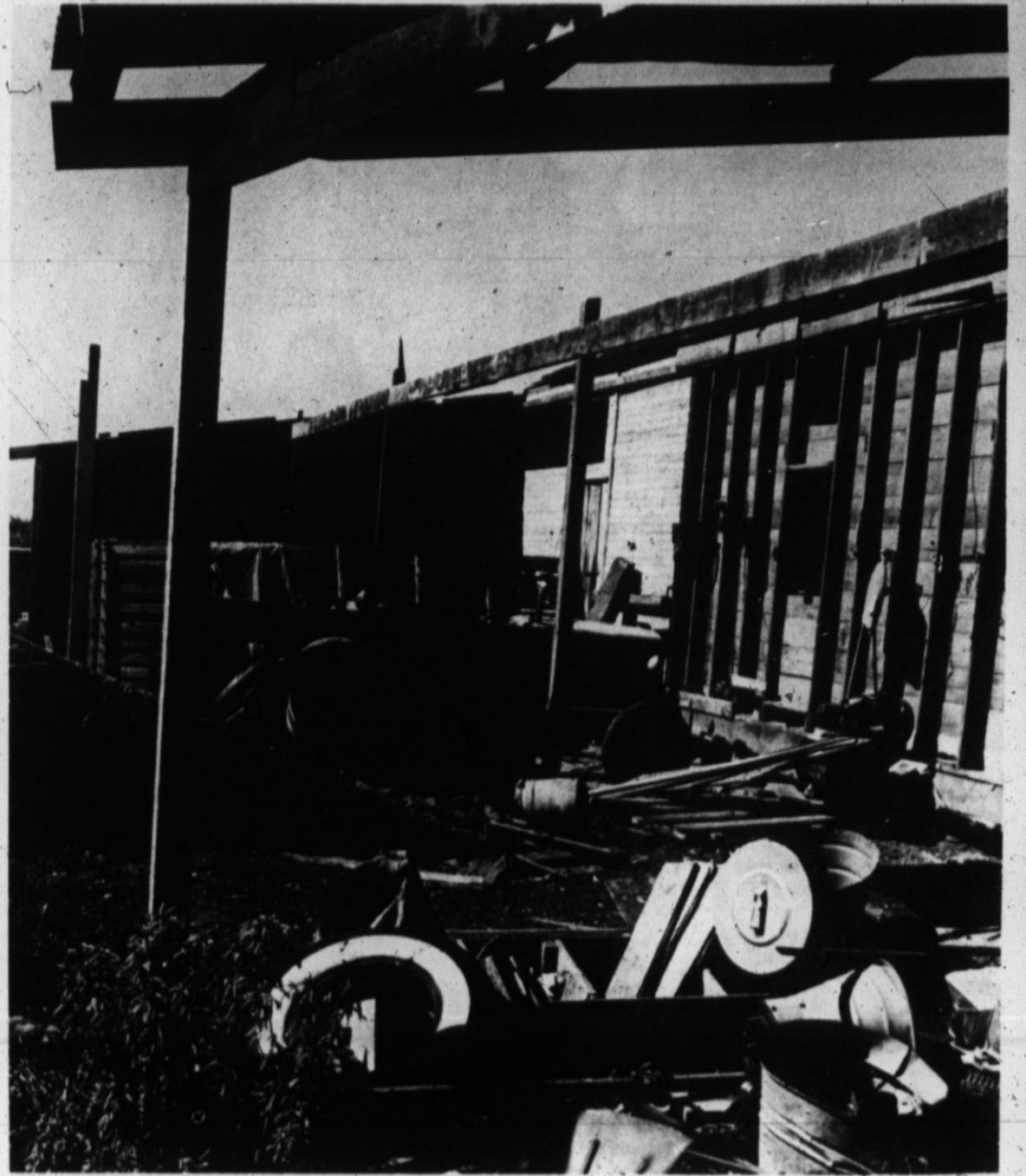
A TOOL SHED ROOF was lifted off of a farm building Wednesday as severe thunderstorms lashed the Deaf Smith County area before midnight. The storm — apparently containing a small twister — struck the John Kalka farm, a mile east of Westway, doing extensive damage to buildings, fences and trees. (Staff Photo)
