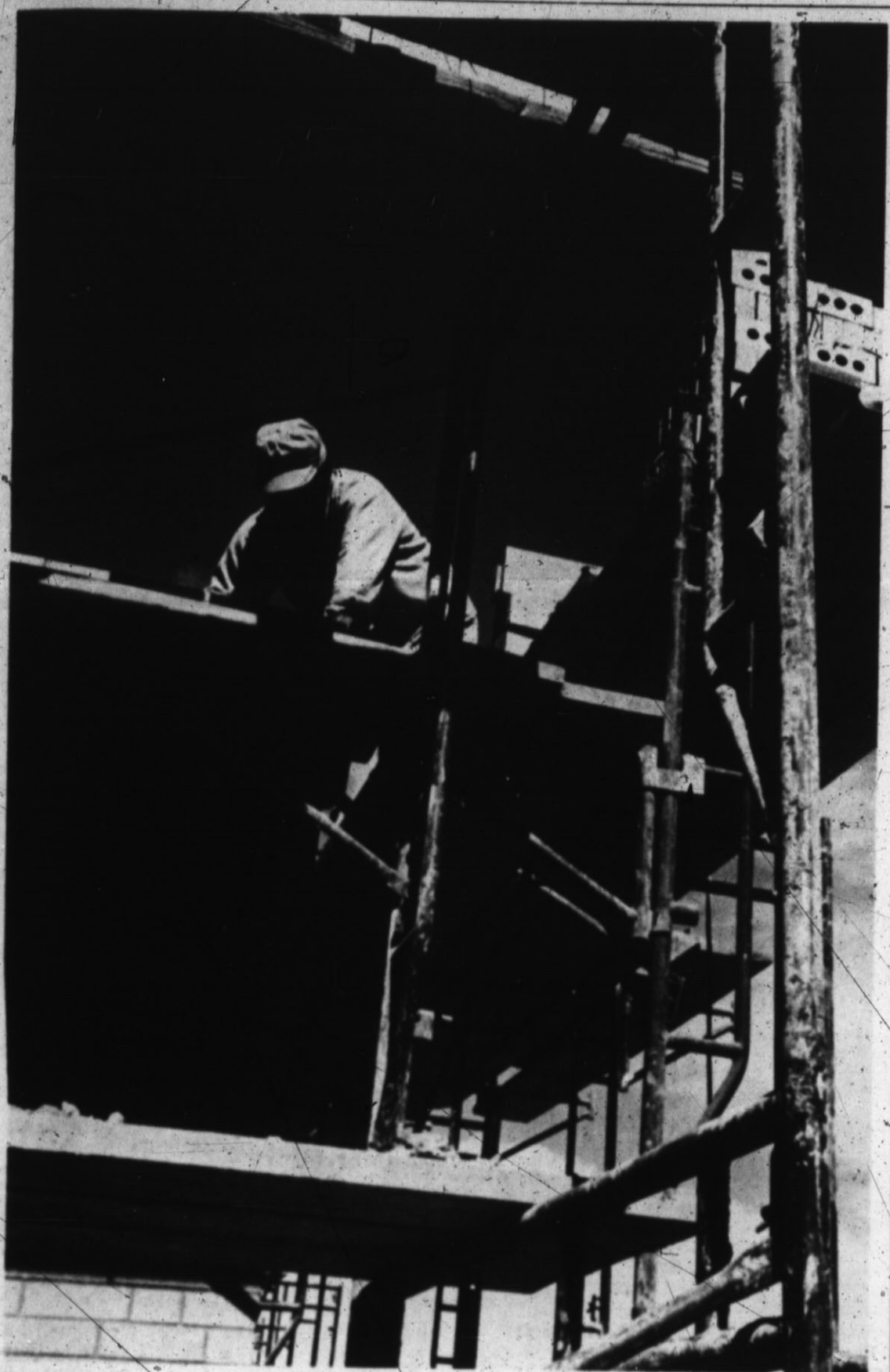
SCAFFOLDING AND BRICK WALLS rise higher and higher as workmen rush to complete the new additions at both Hereford High School and Northwest Elementary School. Both additions are expected to be completed by the time school opens for the 1963 fall term. The addition at the high school will provide more space for home economics department, enlarged science department facilities, additional classrooms, and girls' P. E. facilities. The addition at Northwest will provide more classroom space, office facilities, and a cafeteria. (Staff Photo)
