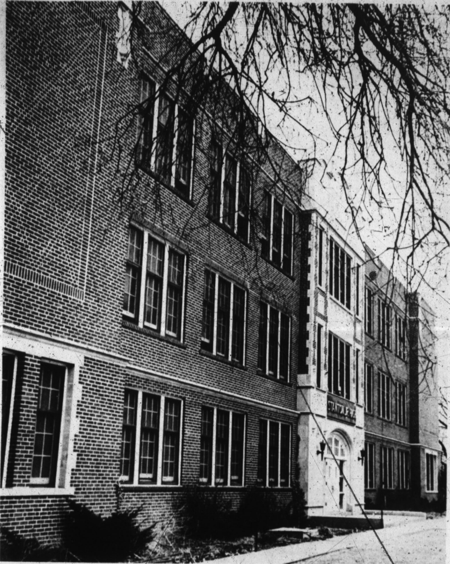
Older portion of Stanton Junior High facilities
