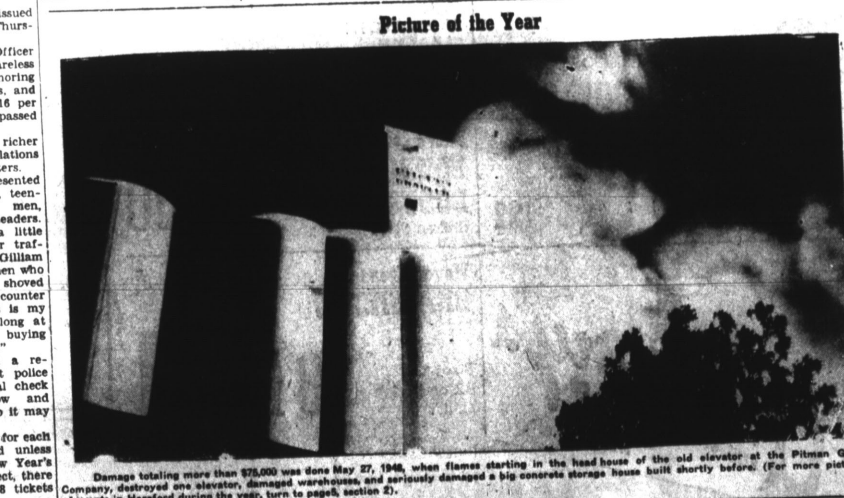
Damage totaling more than $75,000 was done May 27, 1948, when flames starting in the head house of the old elevator at the Pitman Grain Company, destroyed one elevator, damaged warehouses, and seriously damaged a big concrete storage house built shortly before. (For more pictures of events in Hereford during the year, turn to pages, section 2).
