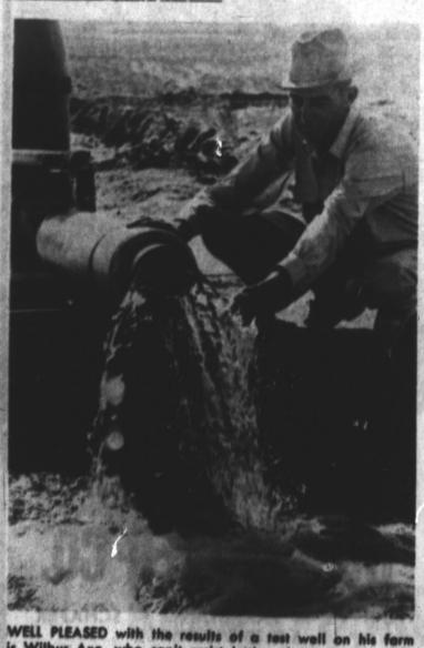
WELL PLEASED with the results of a less well on his farm is Wilbur Axe, who can't resist letting the water run over his hand. The well was drilled as an experimental test, with neighbors offering to defray part of the cost. The well is pumping strong from a strata 800 feet below the surface.
