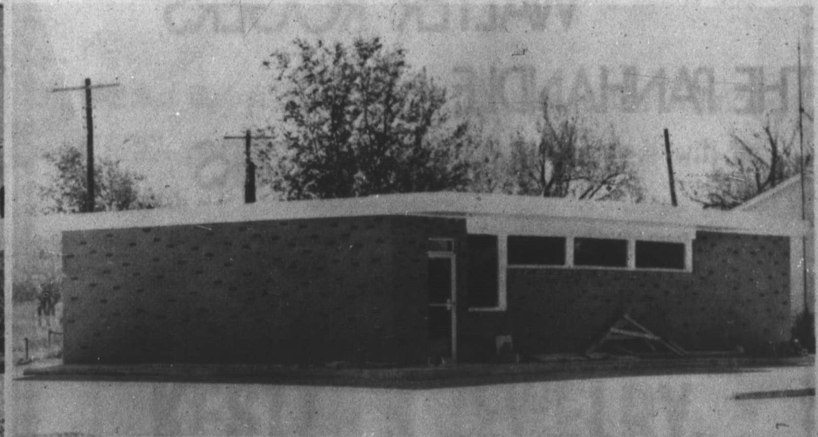
NEW GROCERY STORE — This new building on 25-Mile Avenue will occupy a small grocery store. It is located near Central Elementary School. The store is being constructed by James H. Bradley. The store is rapidly nearing completion.
