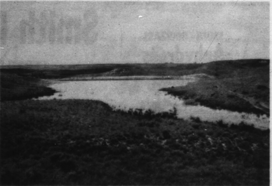
EARTH FILL pond on the J. R. Wheat Ranch. This site was ideal for large storage of work. water with a minimum amount of earth. (SCD Photo)
