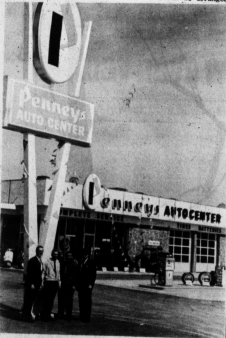
AUTO CENTER — Officials of J. C. Penney Co. pose in front of the Penney's Auto Center at Sugarland Mall Shopping Center, which opened Wednesday. From left are Clete Corlis, manager of Penney's Hereford store; Mel Rogers, Penney's zone auto merchandiser; Ray Stevens, Penney's zone auto service manager; and Tom Homsey, Penney's auto center manager. (Staff Photo)
