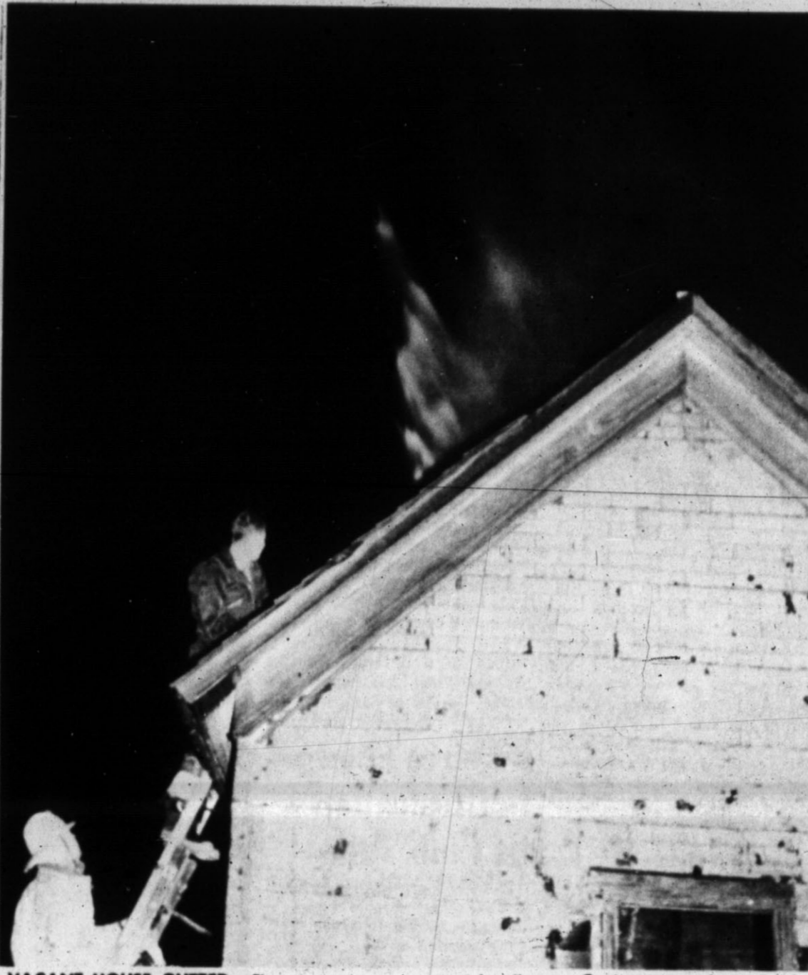
VACANT HOUSE GUTTED —Fireman answered a call to the 300 block of Ave. D late Tuesday night, where a vacant house was gutted by flames. Origin was undetermined. Twenty-three fireman answered the call. (Staff Photo)
