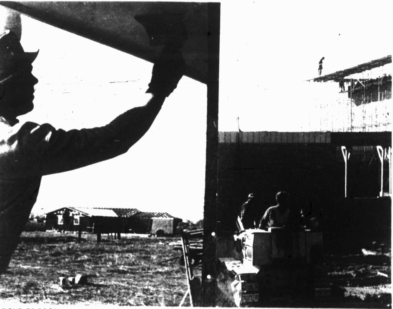
SIGNS OF BOOM — New houses being built virtually in the shade of each other, and construction crews working at the city's newest school addition are signs of a booming economy in Hereford as 1966 gets underway. Bank deposits — as usual — are at an all time high, and new construction here set records for the fourth straight year. Story above, right, outlines prospects for the coming year. (Staff Photos)
