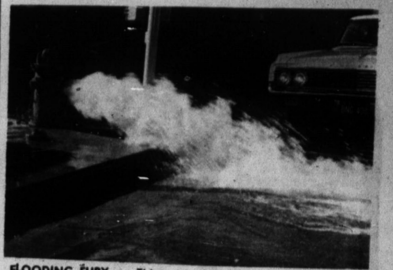
FLOODING FURY — This water hydrant, and many others in Hereford, was opened Tuesday morning for a short time. The purpose of this was to flood the drainage ditches and flush the trash out of the main lines. According to Bill Byers, superintendent of the City's Street Department the purpose was also to eliminate unpleasant odors caused by the cluttered drains. Byers said this is done periodically, depending upon the amount of rain we get.
