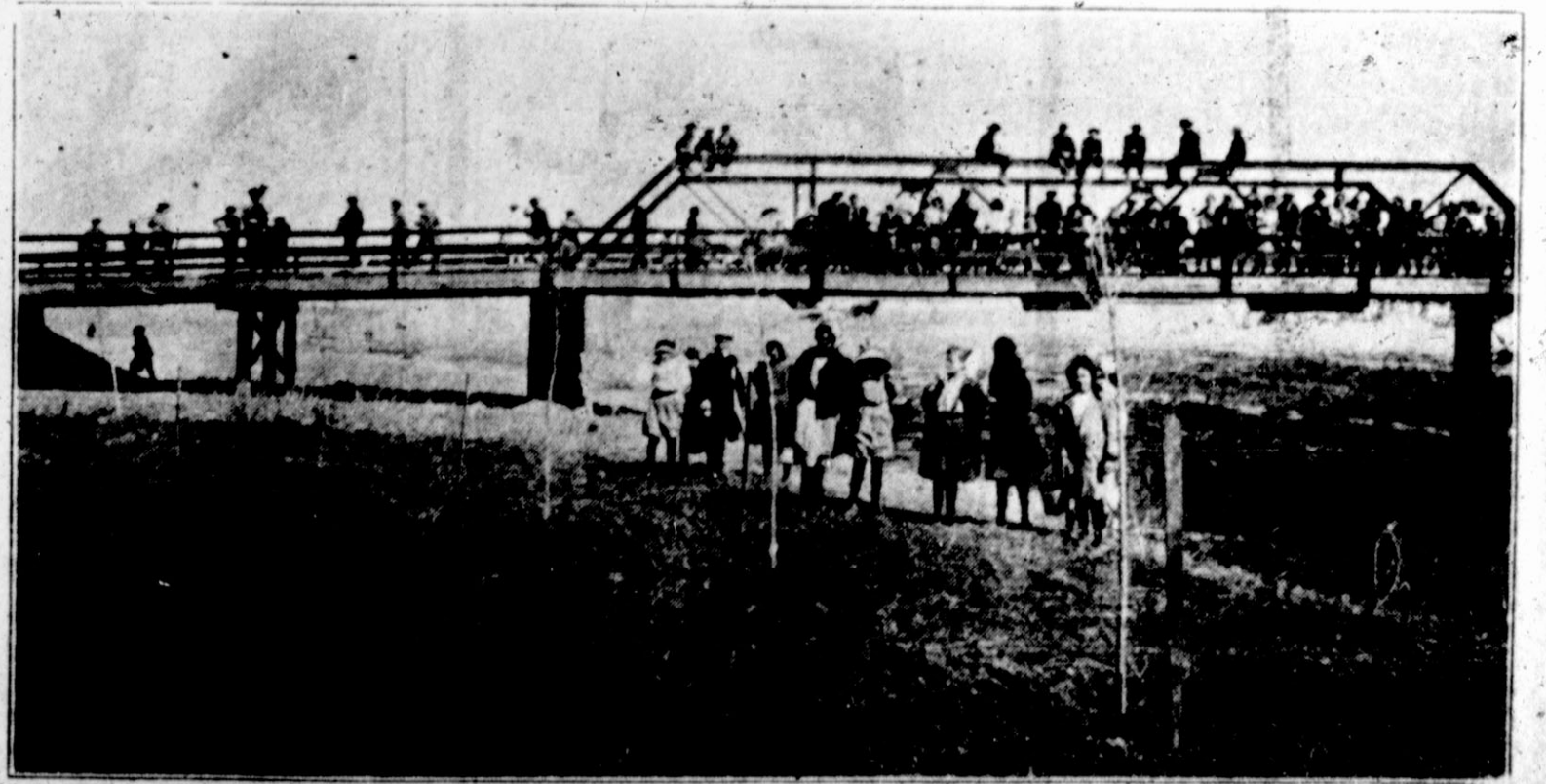
New Bridge Over the Tierra Blanco River. Hereford School Children Who Had Just Finished Planting 600 Trees in City Park, 1908
