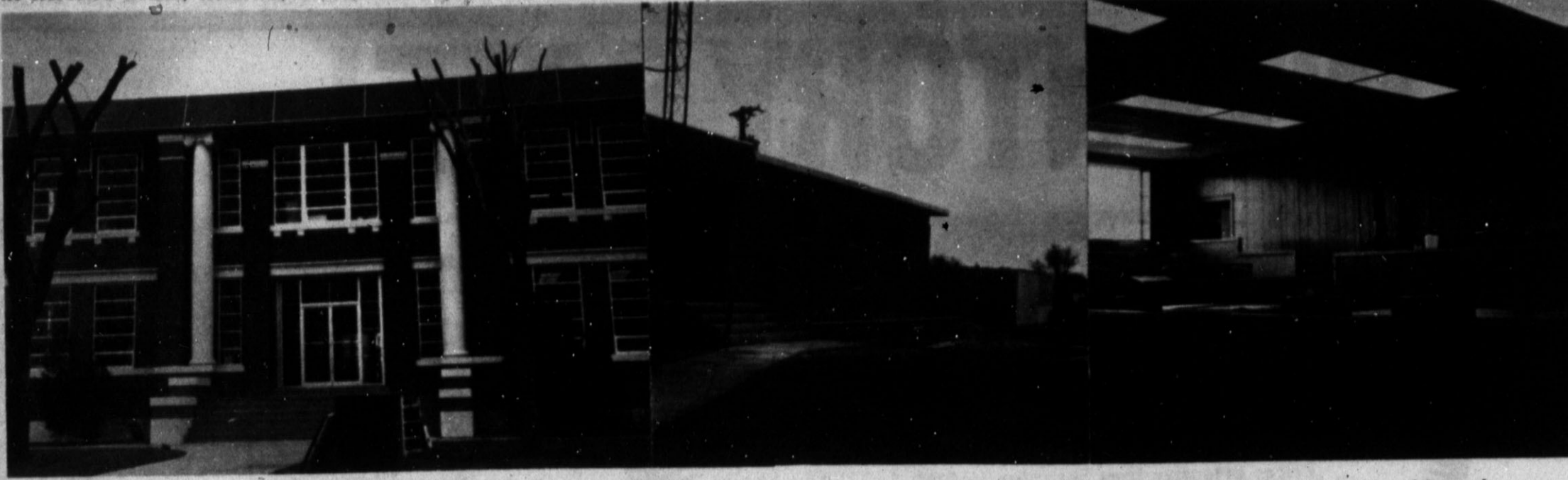
FACE LIFTING NEARS COMPLETION — Renovation of the Oldham County Courthouse at Vega nears completion, with workmen presently waiting on arrival of steel so that the new jail quarters
