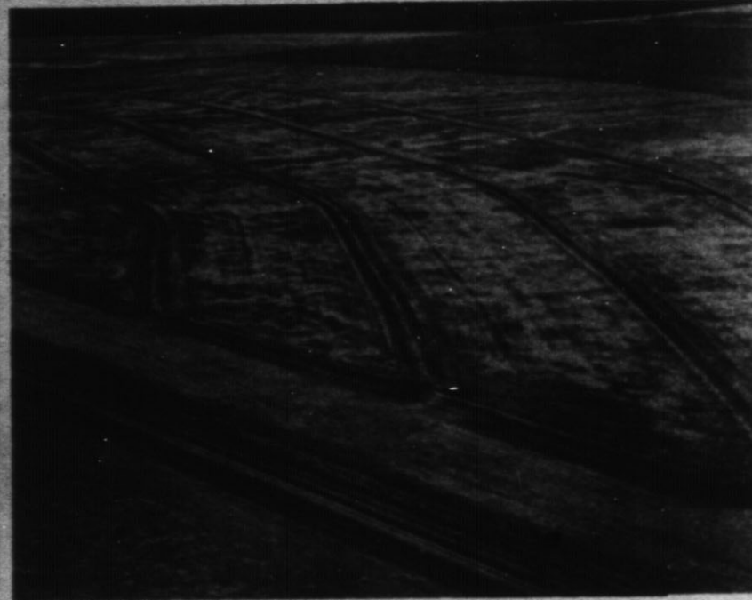
PARALLEL TERRACES — These two aerial photos show the parallel terracing on the Julian Perrin farm from slightly different angles. Perrin has his system draining into a grassed waterway
