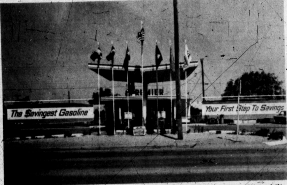
NON-RESIDENTIAL BEAUTY SPOT —The Premier Service Station on Highway 385 was selected non-residential beauty spot for June by members
