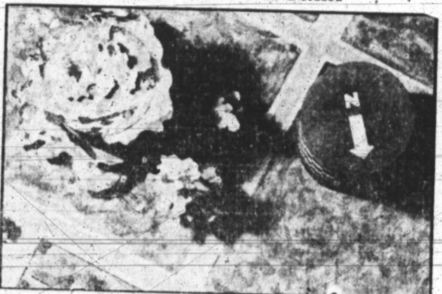
Using concealed light to offset shadows, camouflage experts show how to conceal a huge gas tank from enemy bombers. Shadow angles at various times of the day must be considered to make this type of camouflage effective.
