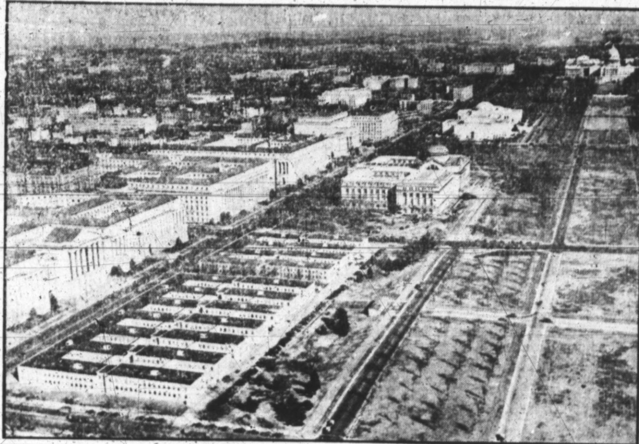
New buildings to house growing government departments have been dubbed "tempo" in contrast to permanent government buildings. Looking east from the top of Washington Monument, visitors see how the squat, box-like temporary buildings change the skyline of the nation's capital.
