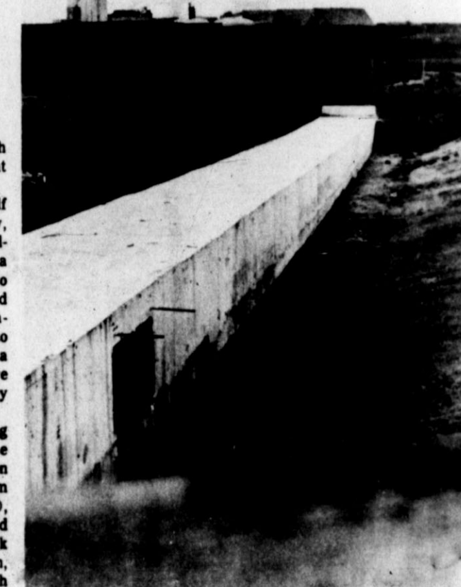
CONSTRUCTION BEGINS —Construction on the new west bound lane of highway 60 began last week with the extension of existing concrete drainage systems to accommodate the new lane. The new addition will add six miles of four-lane highway to existing route.
