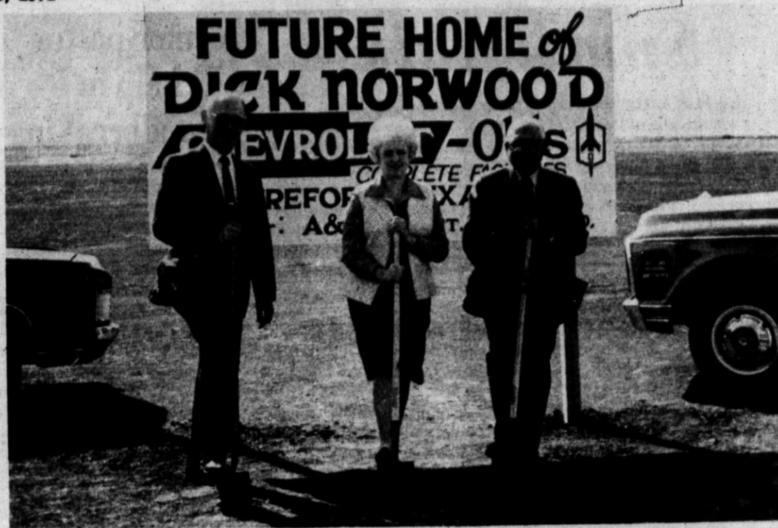
GROUNDBREAKING — Dick Norwood, right, turns a shovel of dirt at the site of the Dick Norwood Chevrolet-Olds dealership which will be built on North 25 Mile Avenue, about one block north of Sugarland Mall, on the west side of the highway. Giving him a hand are Bill Thompson, manager of the Chamber of Commerce, and Mrs. Norwood.
