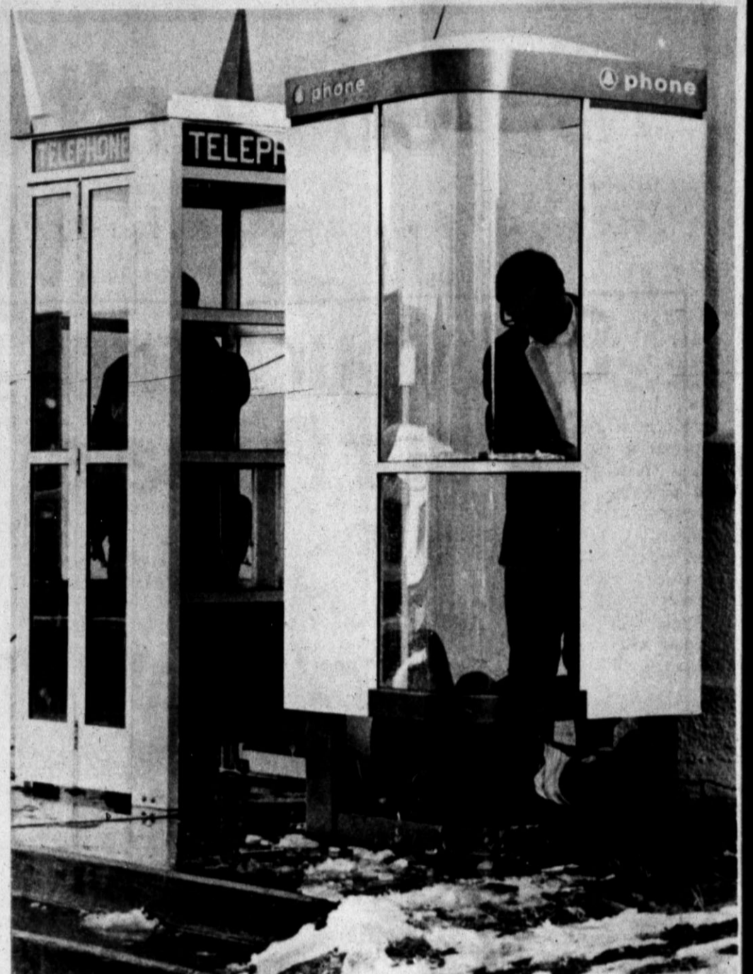
THE OLD AND THE NEW — Southwestern Bell Telephone Company employes, Bob Spaulding and Jack Lloyd, last week installed one of the latest styles in pay telephone booths. The new booth, shown here with its much used ancestor, is now located north of the local telephone office, but will eventually be moved near the front entrance on Miles Ave along with other improvements of decor. The new booth, although it has no door, is quieter and brighter for its users. Photo by Betty Koelzer
