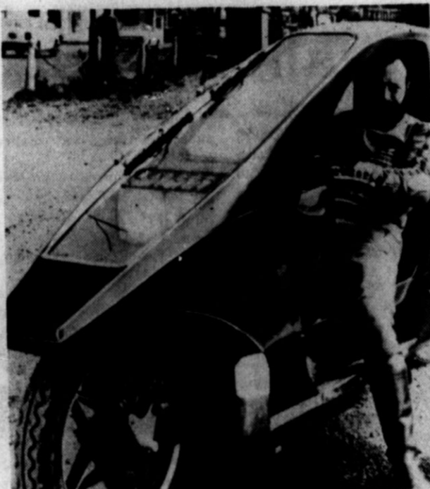
NEITHER WIND, nor rain, nor any other foul weather shall stay the owner of this revolutionary motorcycle from his appointed rounds. Called the "Quasar," the British-built four-cylinder vehicle is powered by a 750cc engine. The cycle's tubular steel chassis is covered by fiber glass and features a roof to keep the driver warm and dry.
