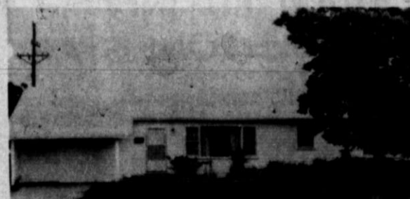
New Roof. New exterior paint. Located in an excellent NW location. 3 Br., 1 Bath, and we'll show you how to own this home.
