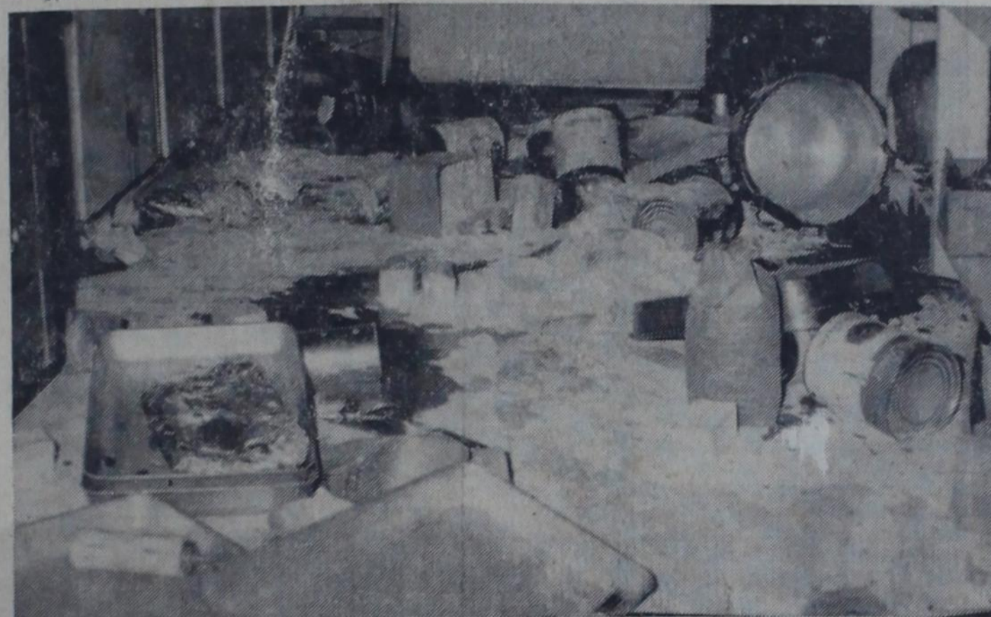
VANDALISM—These views of the Title I, remedial education room at top, and the kitchen of the Rising Star Elementary school lunchroom at bottom show the wreckage done by intruders who broke into the building through shattered windows. Fortunately, according to Supt. Victor Childers and Prin. Weldon Hill, the damage which at first seemed great, will not run more than $1,000 unless two expensive machines cannot be repaired. The damage was discovered by members of the Eighth grade class returning from a picnic Friday afternoon. Two 10-year-old boys were apprehended. Members of the class and their teachers cleared up the mess Saturday and salvaged most of what appeared lost.
