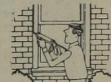
Caulk around doors and windows
