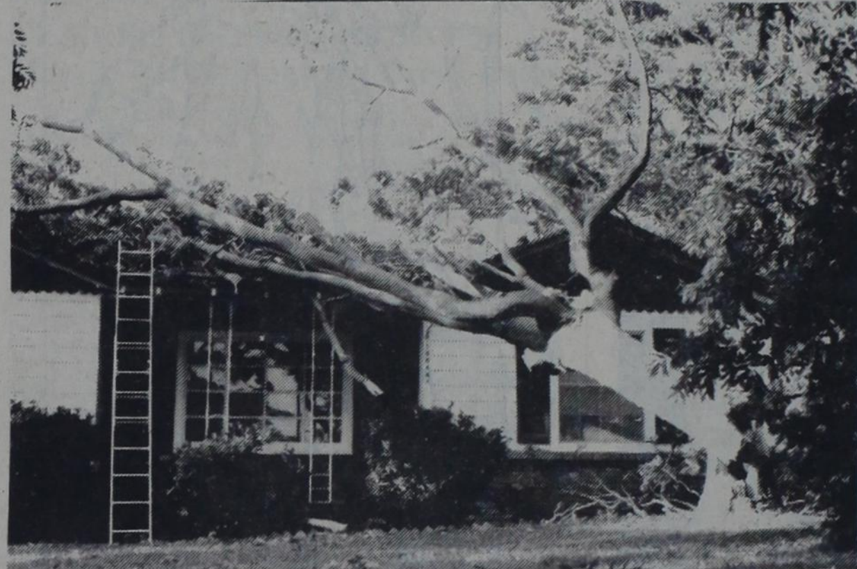
A large tree was blown onto the roof of the home of Ozzie and Ollie Burns Thursday night. Wind gusts were clocked at about 80 mph in Abilene. The tree was diseased in the center.
