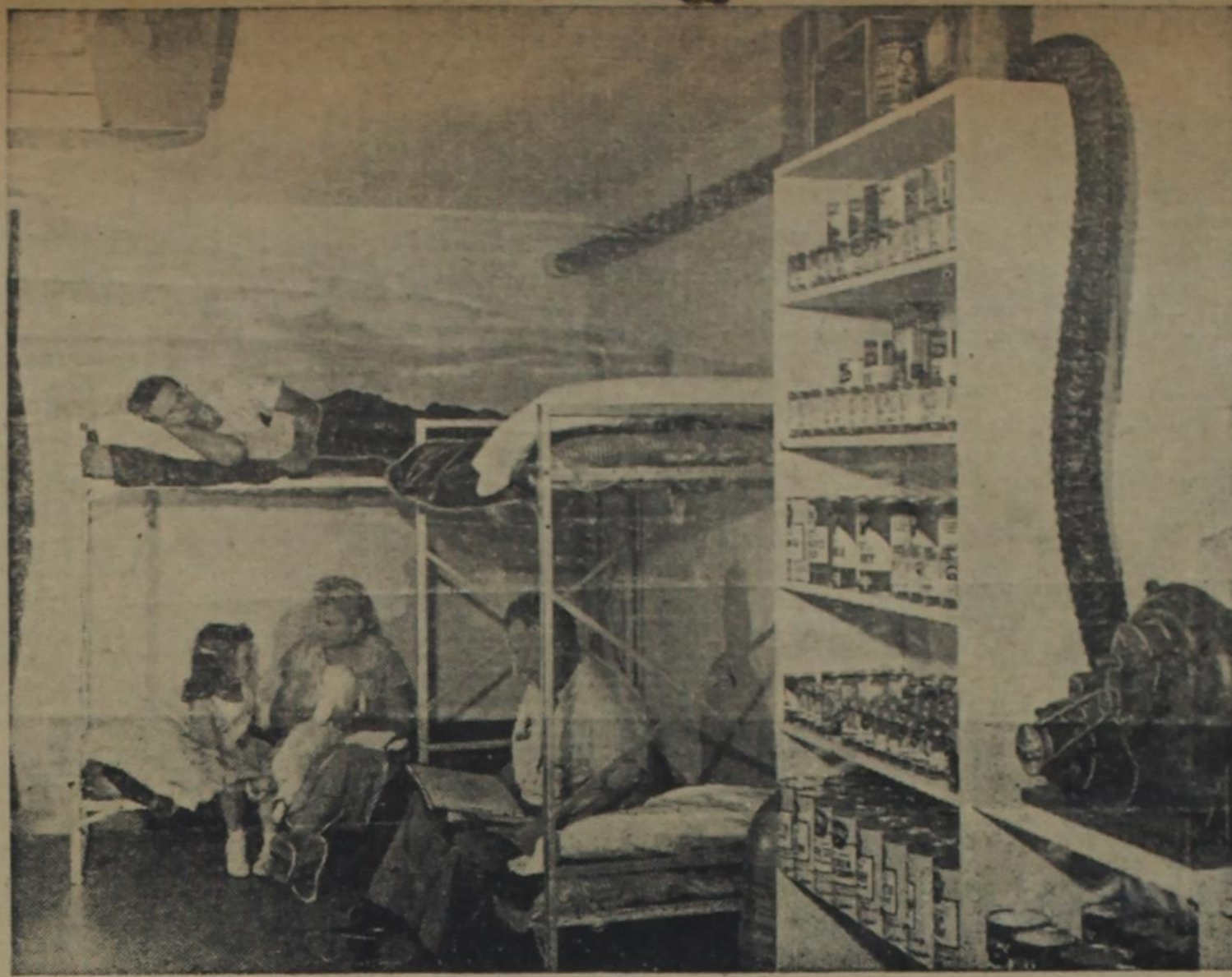
FALLOUT SHELTERS are the best way for rural Americans to protect themselves from a massive nuclear attack which could unleash dangerous radioactive fallout throughout the country. Some of the shelters recommended by the Office of Civil and Defense Mobilization are not as elaborate as this one, which includes an auxiliary generator and an electric air filtering and ventilating system. However, all recommended shelters should include the basic features shown here—a place to sleep; food, water and medical supplies, and at least eight inches of concrete as an equal weight of other materials for shielding the shelter against fallout. Free designs may be obtained by writing to OCDM Rural Civil Defense, Battle Creek, Mich. (OCDM Photo)
