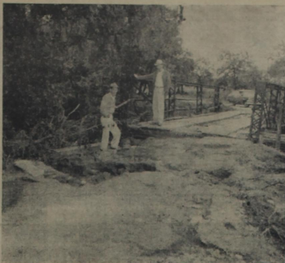
Harold Garrett, Cross Plains livestock farmer and John Lee, SCS Conservationist, Rising Star, survey damage to Callahan County road bridge left by October 1957 flood in Turkey Creek. A similar bridge in Brown County was completely destroyed by this flood.
