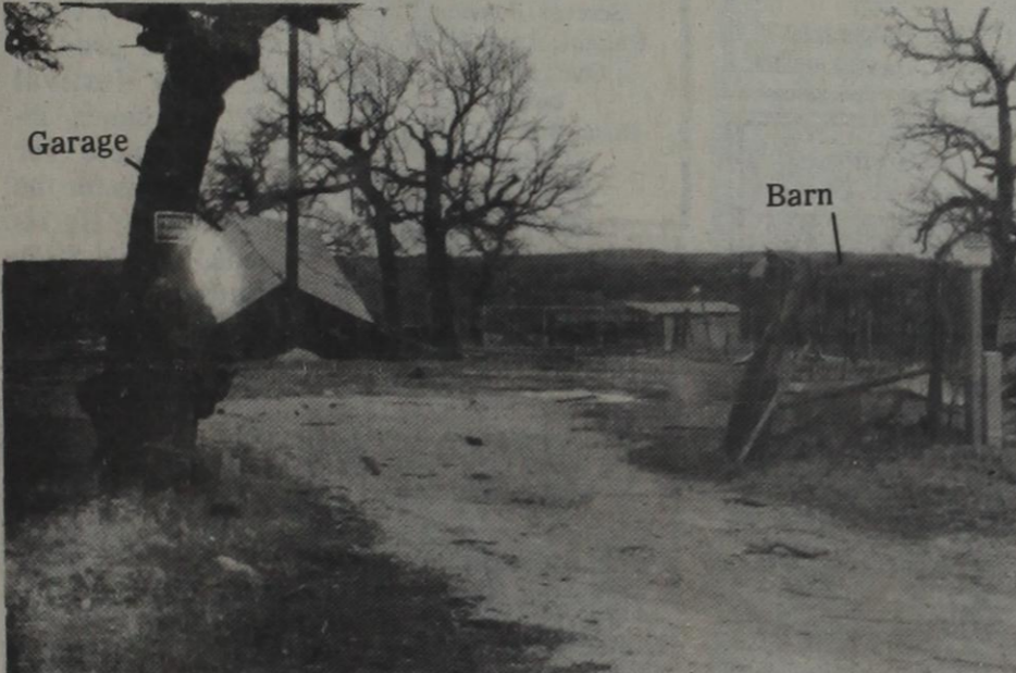
The garage collapsed and the roof was torn from the barn as the tornado moved down from the clouds.
