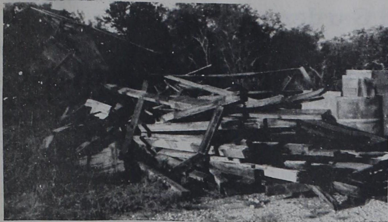
The above building was reportedly in the process of being torn down last Thursday when it collapsed causing injuries to a Sipe Springs man who was inside the building. He died in a DeLeon Hospital reportedly from the injuries.
