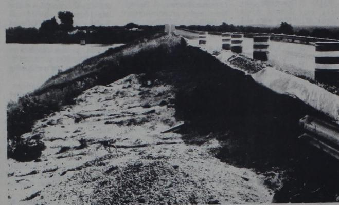
Dam slippage-erosion is still very visible at Lake Leon dam.
