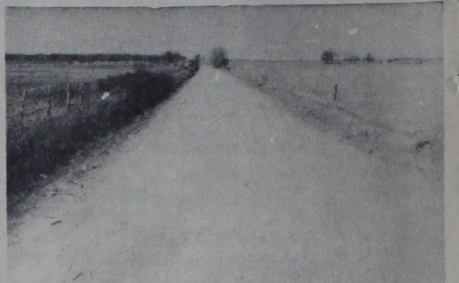
Entrance to the new dump ground - the road is bordered on the right by landowner Wilbur Caudle and on the left by Ray Agnew.
