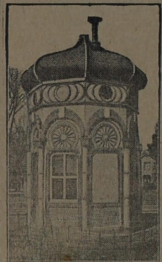
Looks Like a Mosque but is Flagman's Shelter.
