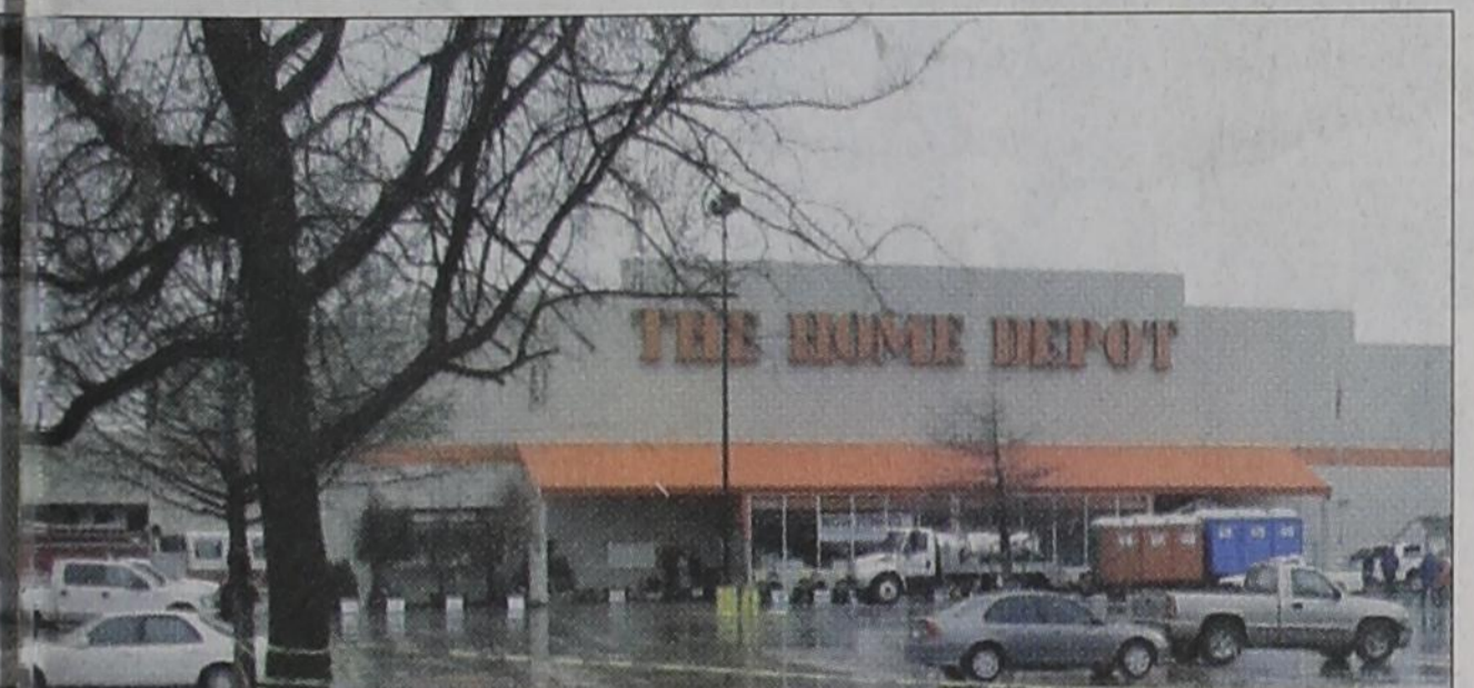
Water main that feeds the indoor sprinkler system at the Rockwall Home Depot broke during the night of March 9, causing flooding within the building and leading to an indefinite closing of the home improvement store. Stephen Holmes, Home Depot spokesman from Atlanta, Ga., said a structural engineer has inspected the building and found it to be secure. Employees and workers are cleaning up the mess, but Holmes would not give a reopening date as there was significant product damage that has not yet been processed. No one was in the store at the time of the incident.
