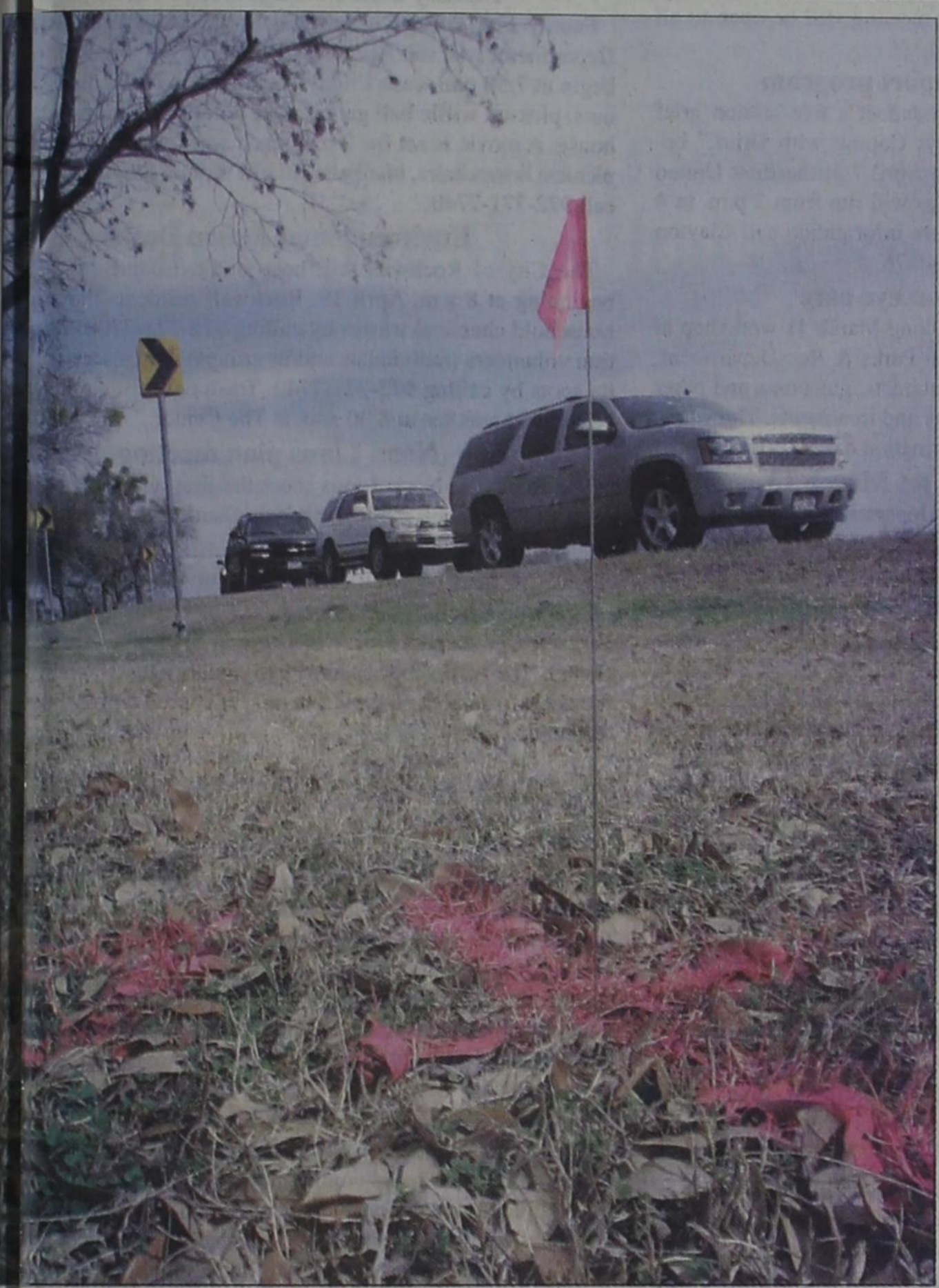
Marking FM 740 (Ridge Road) south of IH 30 this week reminds motorists of future road expansion as part of last year's road improvement bond issued approved by voters. Staff Photo by Tim Burnett
