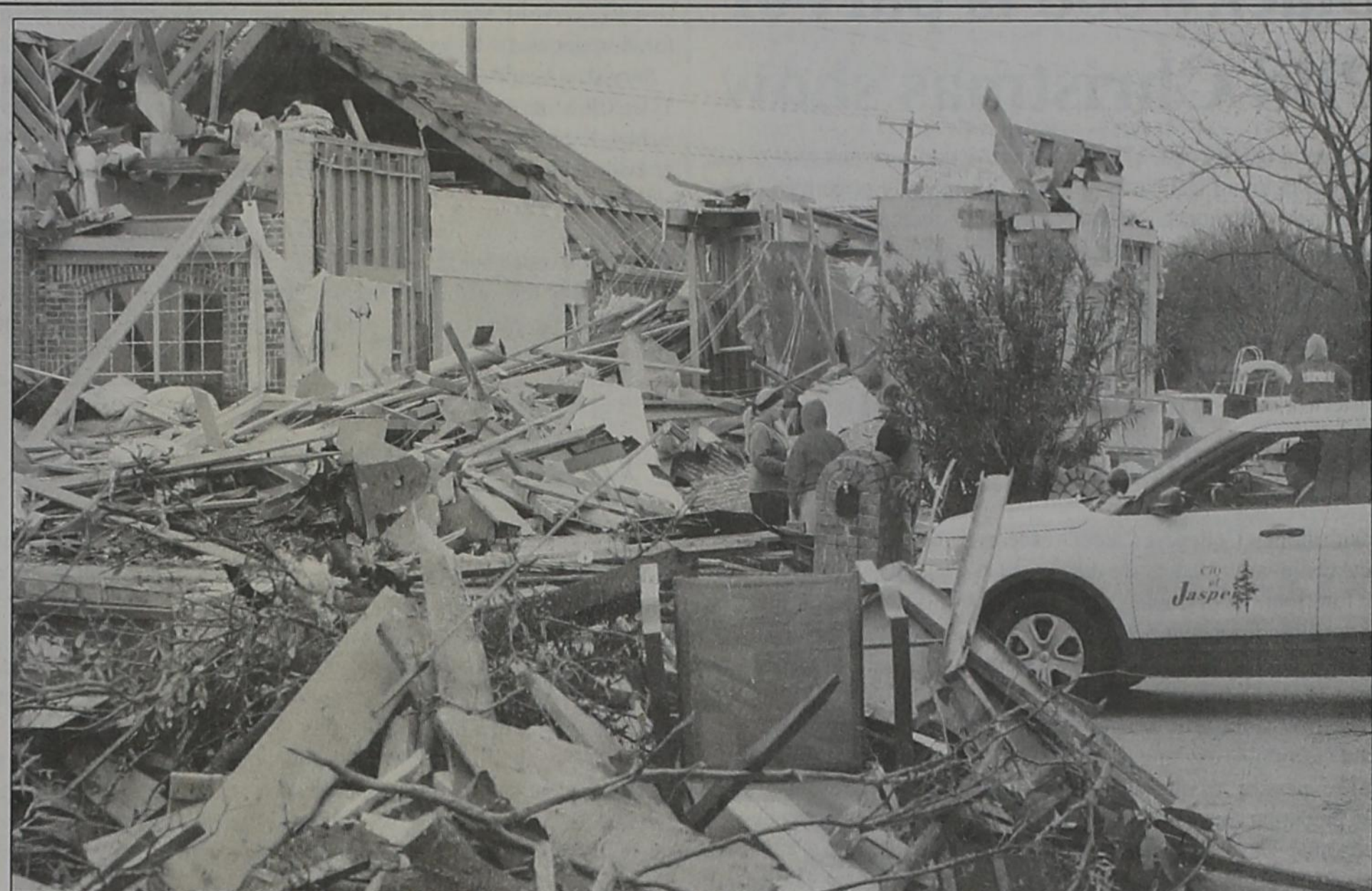
Mike Collier, Chief Building Inspector for the City of Jasper, Texas, (shown in the car), assists in assessing structural damage caused by the Sat. Dec. 26, 2015 tornadoes that destroyed many homes in a housing development off Dalrock Road in Rowlett. Representing the Building Officials Association of Texas, Collier left home at 3:00 a.m., Mon. Dec 28 to begin the assessment process and assist as needed. Collier also assisted in the recent flood damage assessment and relief efforts in Wimberly, Texas. Shown at front is a home that was reduced to a large mound of rubble.
