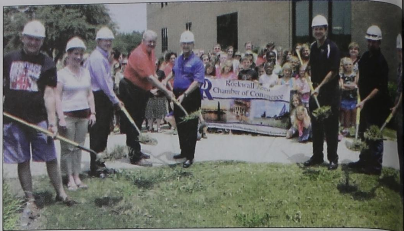
Heritage Christian Academy recently broke ground on a three-phase building project, with the first phase, a math and science initiative, scheduled for completion prior to the start of the 2012-2013 school year. Pictured at the groundbreaking are, from the left, Mike Harmon; Jennifer Hill; Robert Harter, assistant headmaster; Ron Taylor, headmaster; Rusty Wallis; Richard Henson; Craig Cooper; and Oliver. Also shown are board of trustee members for HCA.
