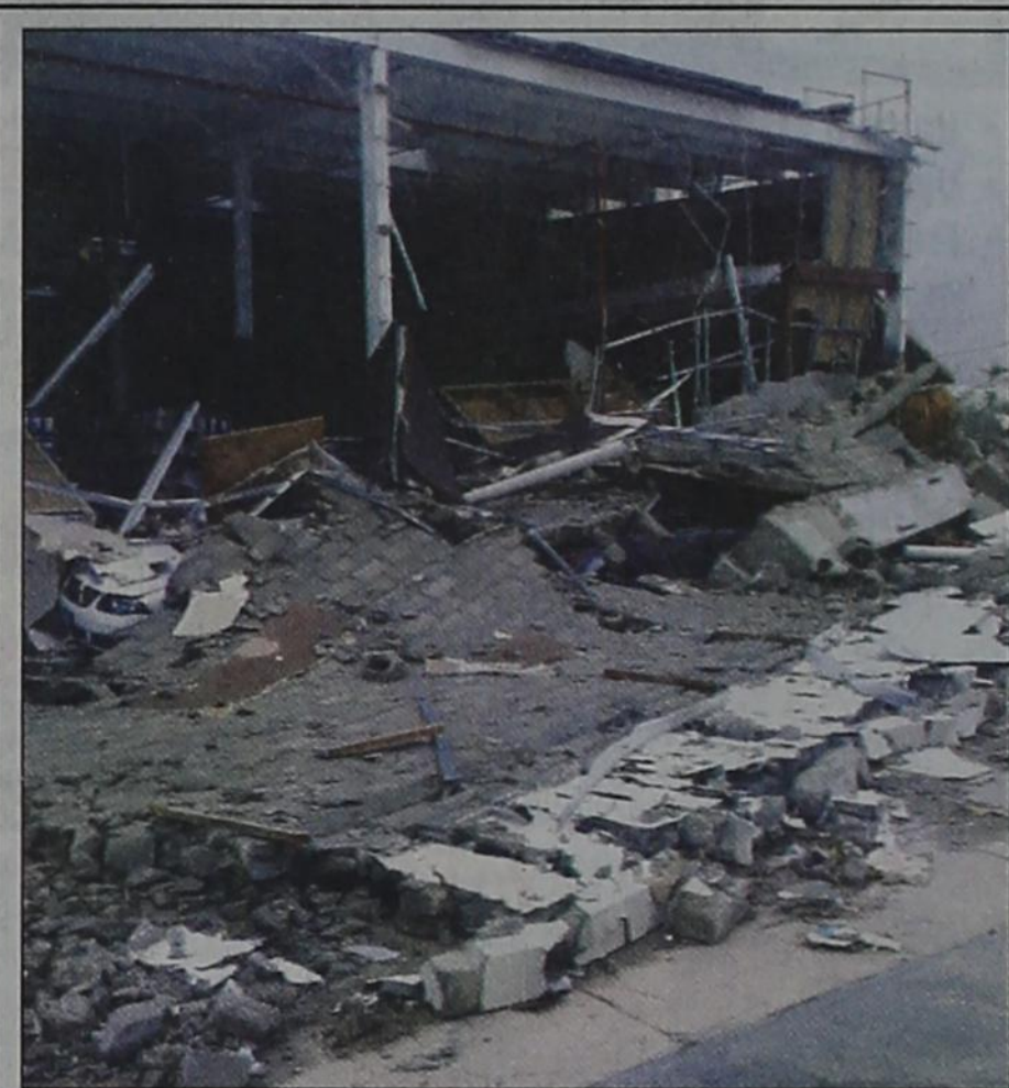
This is the remains of a home improvement store after Hurricane Odile ravaged Los Cabos, Mexico, on Sept. 14.
