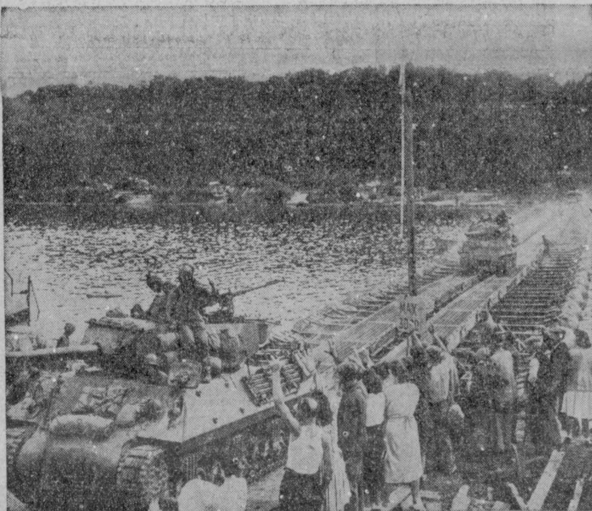
CROSSING THE RIVER SEINE —Hastily constructed bridge replacing one destroyed by retreating Germans, carries Allied tanks and crews across river Seine. French civilians cheer as friends wind way over pontoon bridge to continue drive against enemy.
