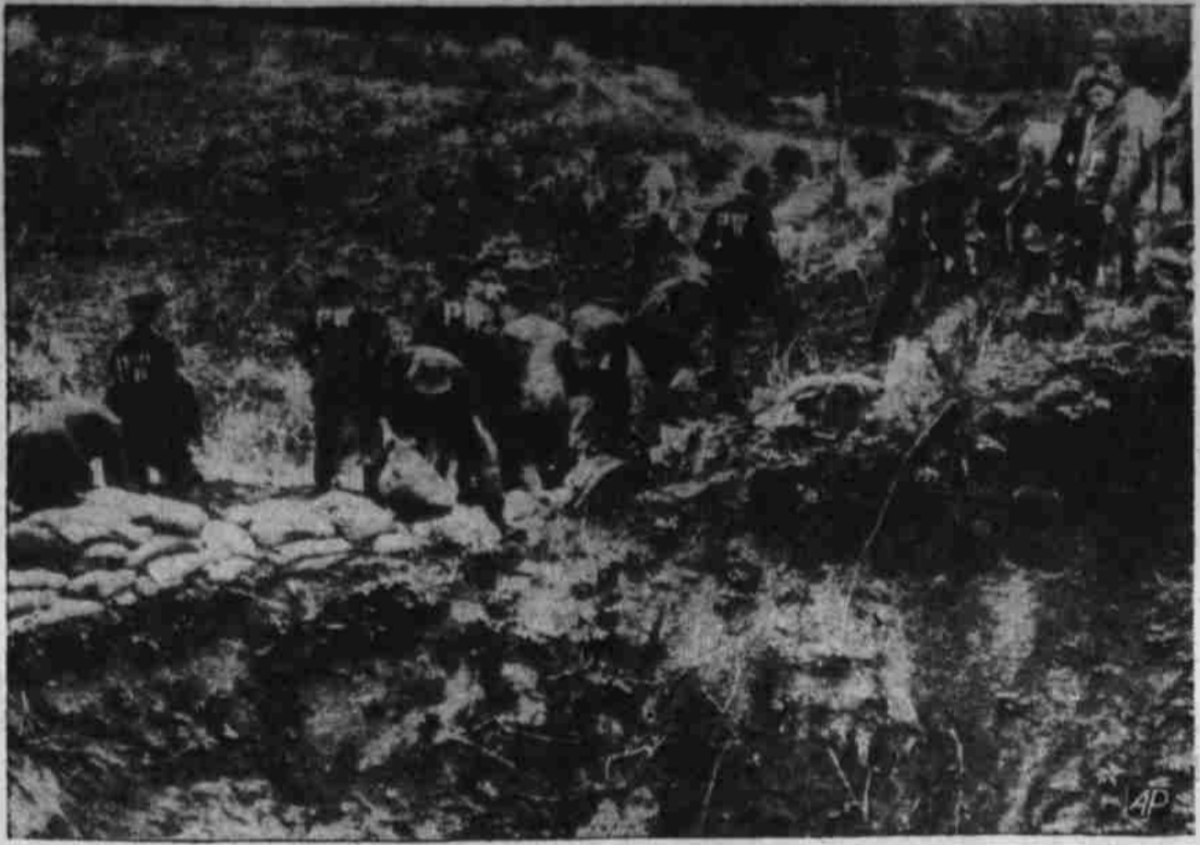
Axis Prisoners Sandbag Levee— Acting under emergency authorization, Axis prisoners of war were used by United States army engineers to sandbag crevasses on the Mississippi river south of St. Louis last week. The "PW" appearing on the back of their jackets identify them as prisoners of war.
