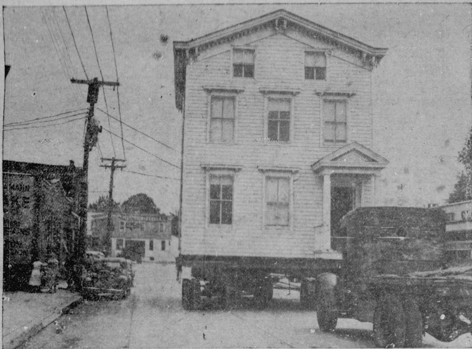
OFF TO A NEW LOCATION —While being moved by truck to a new location in Hempstead, N. Y., the height of this old three-story house caused line-men to relocate wires, allowing the tall building to pass through a busy section of the town. Traffic was rerouted as wires along the street had to be taken down and then replaced.
