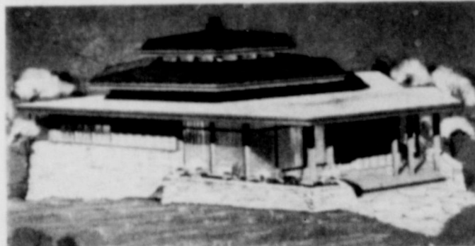
ADMINISTRATION --This building will serve as Camp Rio Blanco office, living quarters for the director, assistant, waterfront staff, and others.
