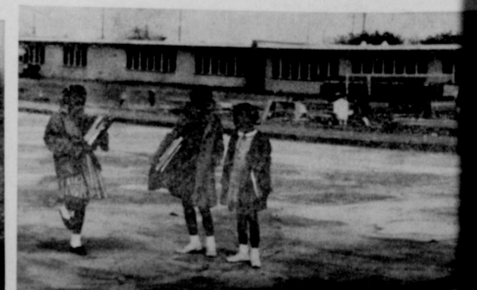
POSSIBLY SKIPPING IN ANTICIPATION of the fun ahead, three students, of Evans school, 1035 East Geneva in Slaton, cross the newly-erected of the large gymnasium under construction there. Steel is being delivered, and completion of the 12,240 sq. ft. building is scheduled within days.
