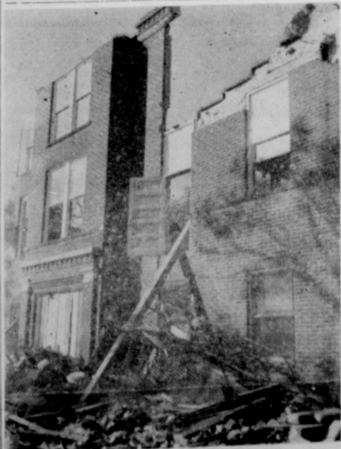
"Decapitating" of the Slaton City Hall preceded remodeling
