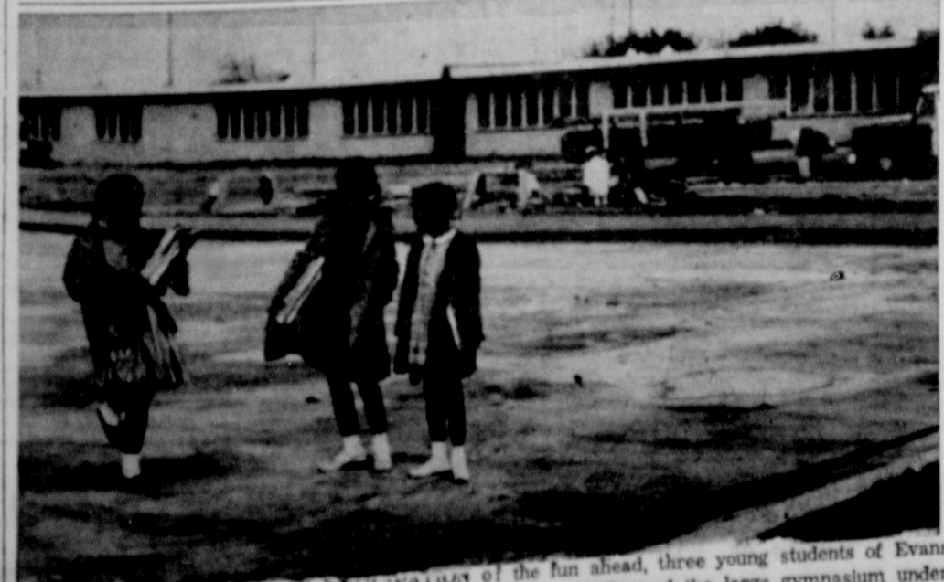
POSSIBLY SHUFFLING IN ANTICIPATION of the fun ahead, three young students of Evans school, 1035 East Geneva in Slaton, cross the newly-poured floor of the large gymnasium under construction there. Steel is being delivered to the site, and completion of the 12,225 sq. ft. building is scheduled within 40 working days.
