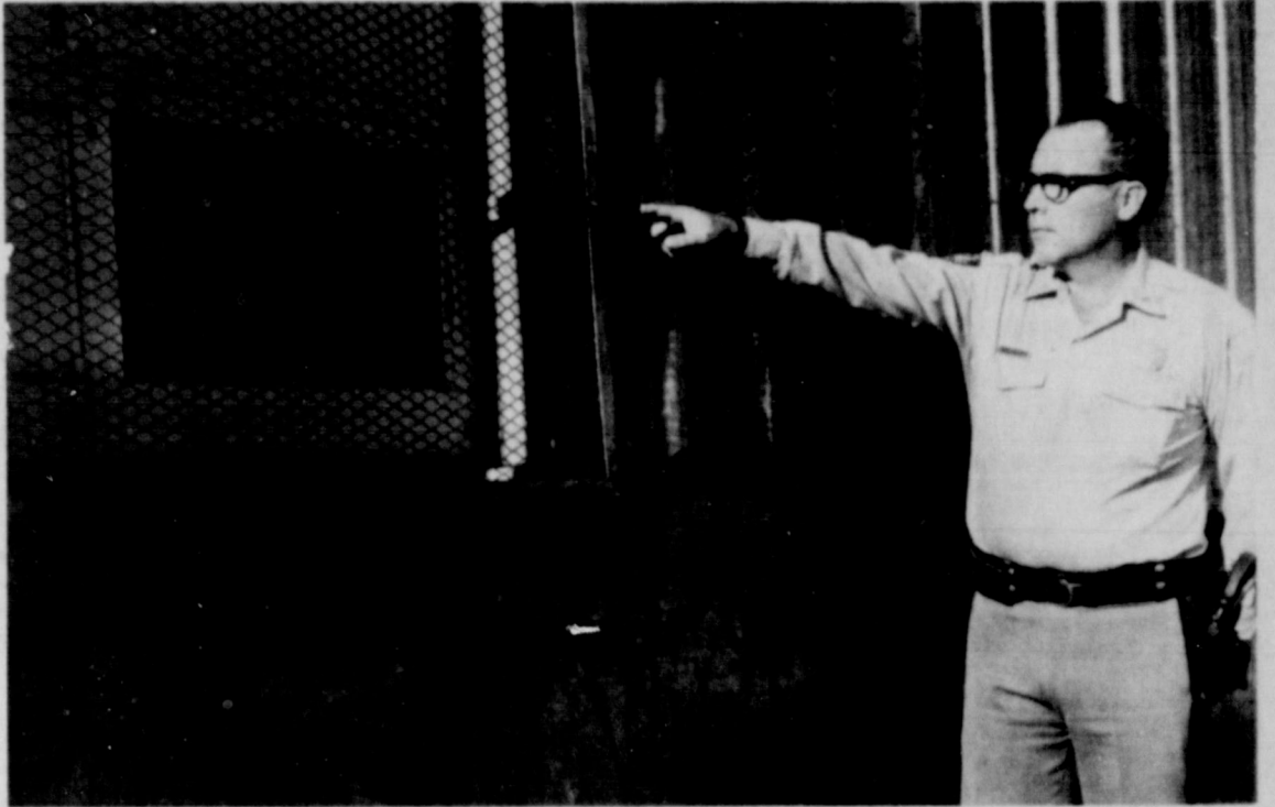
WHERE BURGLARS ENTERED--Slaton Police Officer Darrell Denny points to the hole made in a door where burglars entered the Hestand Wholesale Grocery Warehouse during the night Monday. The screen cover first was piled loose. The intruders took an estimated $600 worth of cigarettes.
