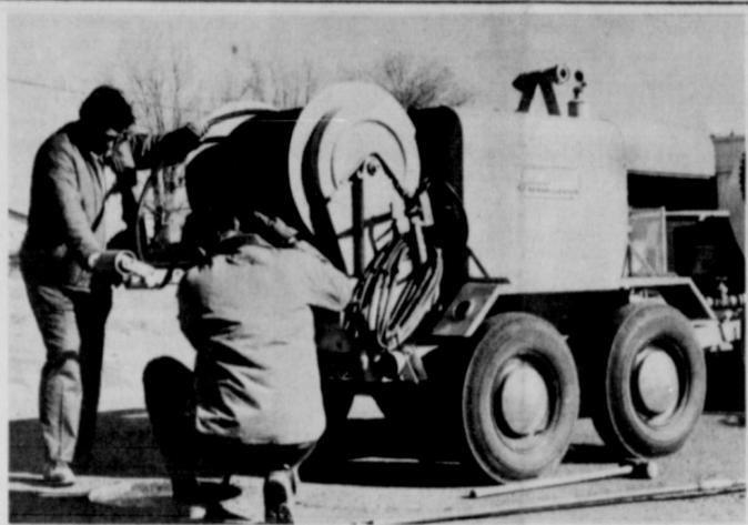
**NEW CLEANING MACHINE** -- City employees Jim Powell and Melvin Norwood are shown here operating the city's new sewer cleaning machine capable of reaching 500 feet into a sewer line and flushing it out. The machine greatly speeds up the process of freeing sewer lines with a minimum of trouble. The machine and water tank on the truck cost a total of about \$5600 and was bought with revenue-sharing funds. (SLATONITE PHOTO)
