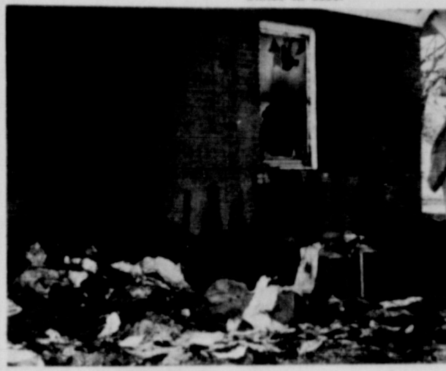
FIRE DESTROYS HOME -- A blaze discovered about 3:30 a.m. Tuesday gutted the home of the Ray Wilson family on U.S. 84 bypass. Cause of the blaze was uncertain. The family was at home at the time, but no one was injured. The fire was out of control before firemen arrived. This is a view of the exterior taken several hours after the blaze. (SLATONITE PHOTO)
